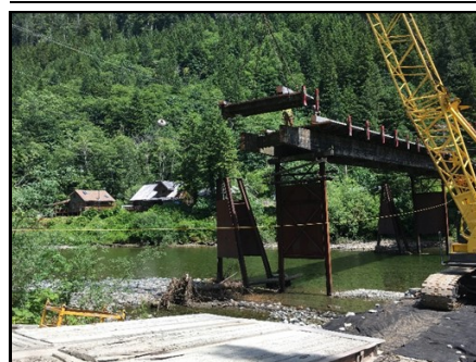
Crews removing the Bridge Deck
