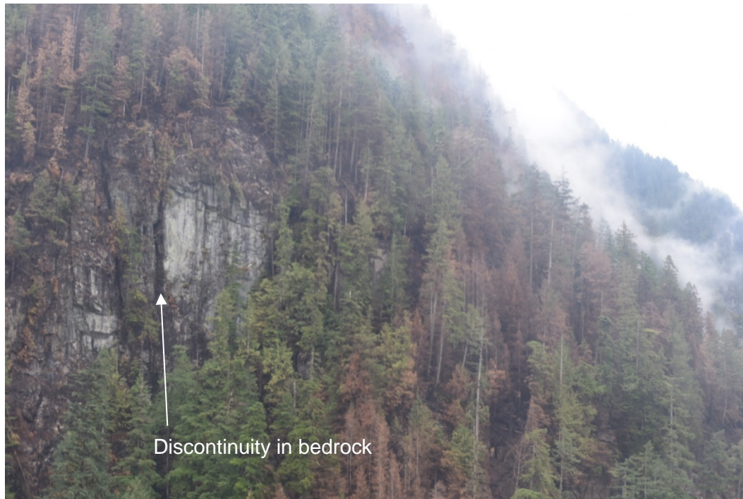
Figure 4-2. Photograph of a dilated bedrock discontinuity upslope of Ferris Road exposed by fire.
