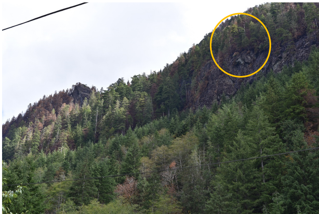
Figure 4-3. Photograph of previously concealed (fully tree-covered) outcrop with overhanging blocks. Photograph by BGC, September 13, 2018.
