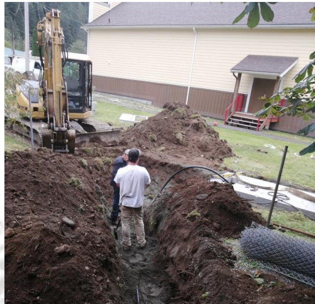
Figure 9 - Trenches excavated to lay power cables to the buildings
