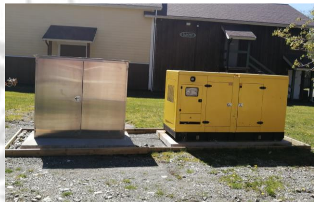
Figure 10 – Completed Generator Project
