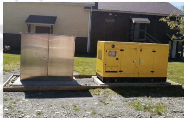
Figure 10 – Completed Generator Project
